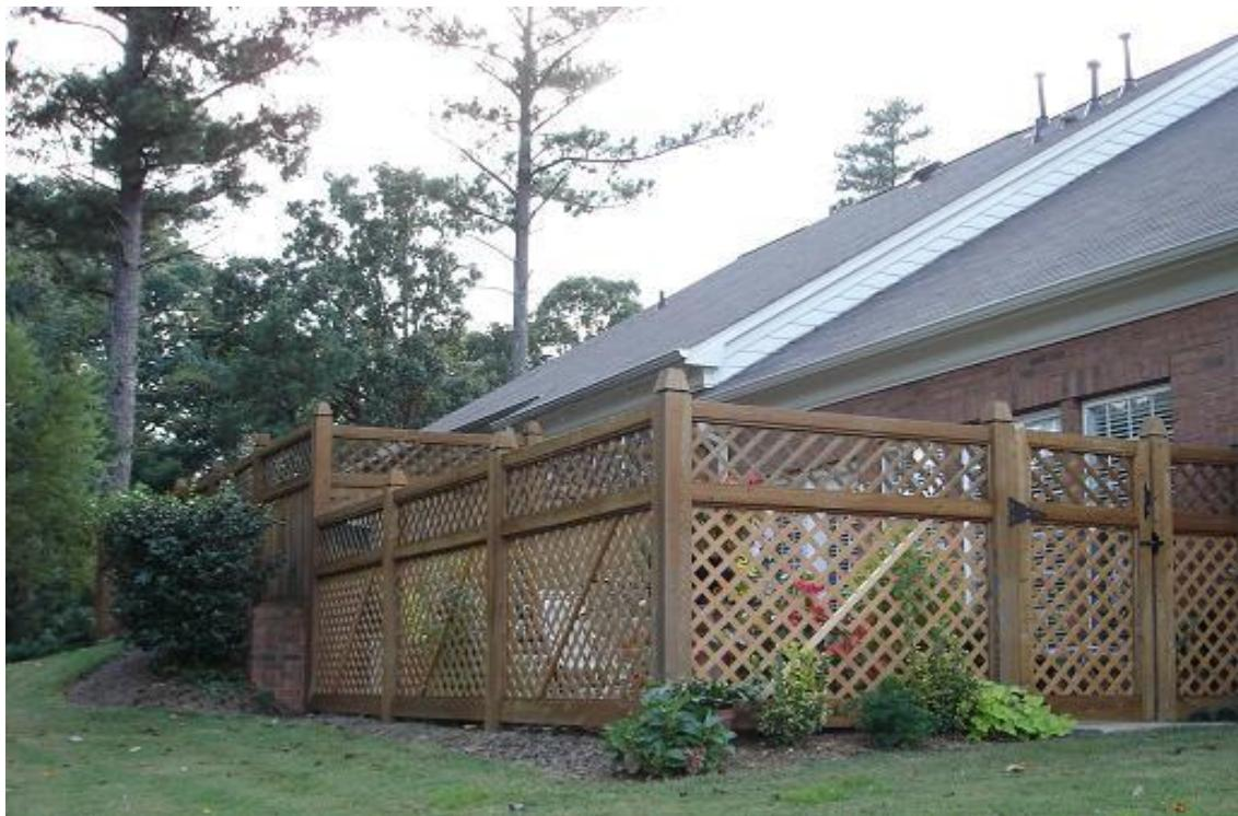
This picture shows the detail of the diagonal brace to give the lattice panel better rigidity: (Not required with the  $\frac{3}{4}$ " lattice.)
